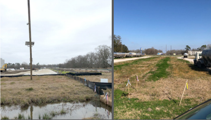
Crews safely work on pipeline construction projects throughout West Baton Rouge.
