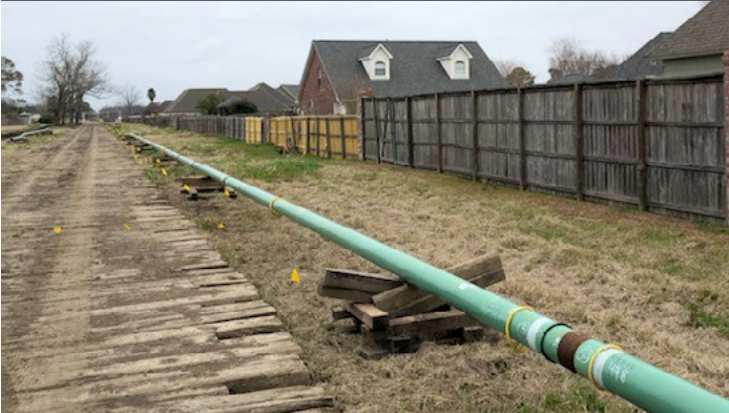
ExxonMobil Pipeline crews working on pipeline installation near the Antonia Plantation Estates subdivision in Brusly, Louisiana.
